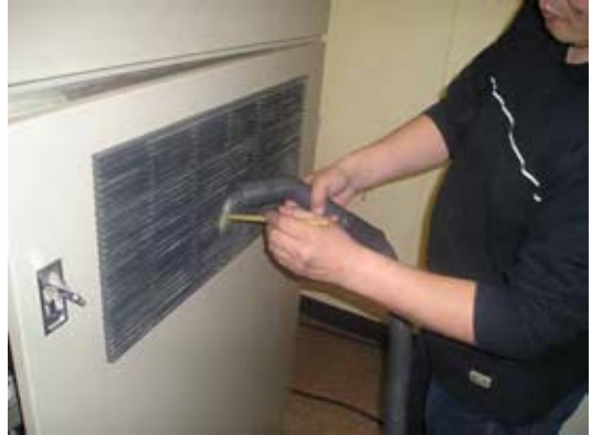
Cleaning of air filter of rear doors
