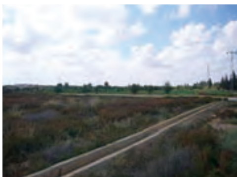
A concrete farm ditch
