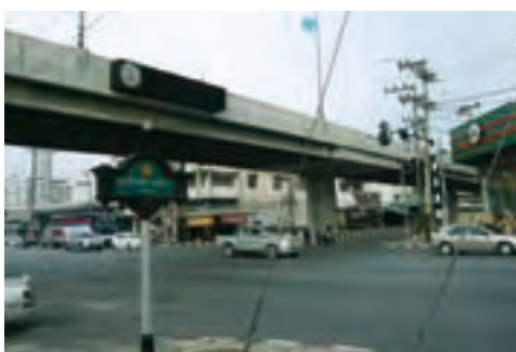
An overpass constructed
