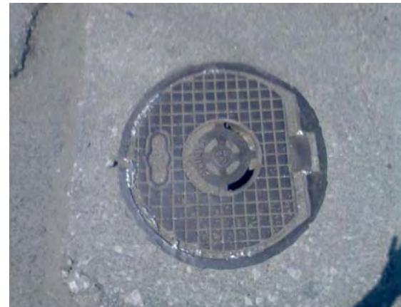
Some of the manholes cannot be opened as they are covered by new layer of asphalt or permanently welded, as shown in the picture below.
