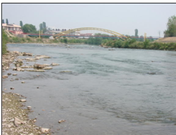
Point (A) UN Bridge (Vardar River)
