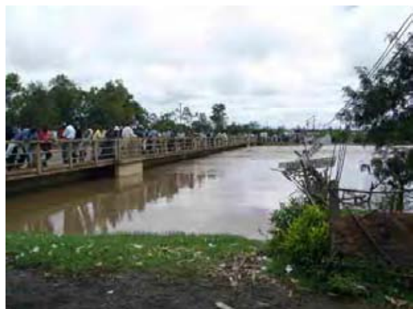
Plate 3 Ahero Bridge during Flood
