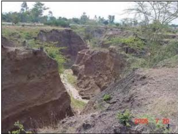
Plate 4 Heavy Soil Erosion
