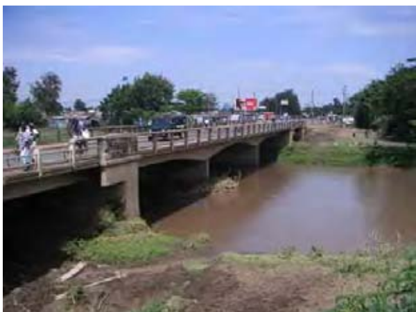
Plate 2 Ahero Bridge at dry season
