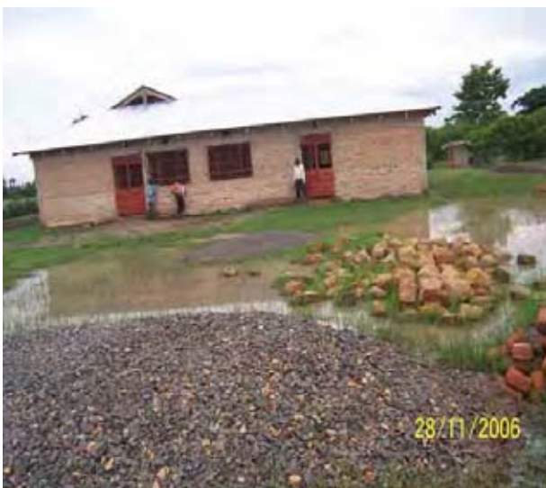
Plate 7: A submerged school during floods
