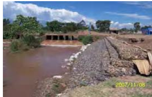
Plate 7: Rehabilitated river bank at Nyamasaria (restricted area is 150m downstream from the bridge)
