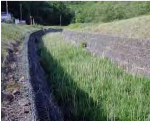
Figure 3.7 Image of Riverbank Protection by Gabion Mattress (in Japan)
