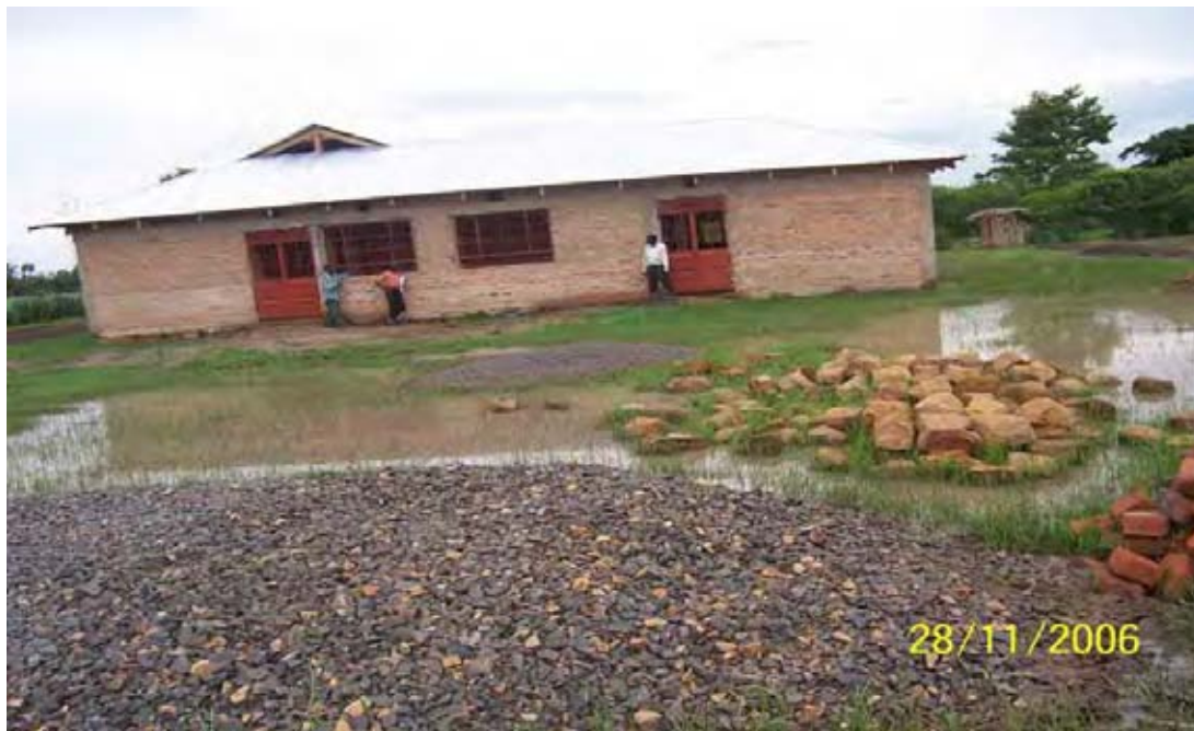
Plate 19 A submerged school in Nyando River Basin during floods
