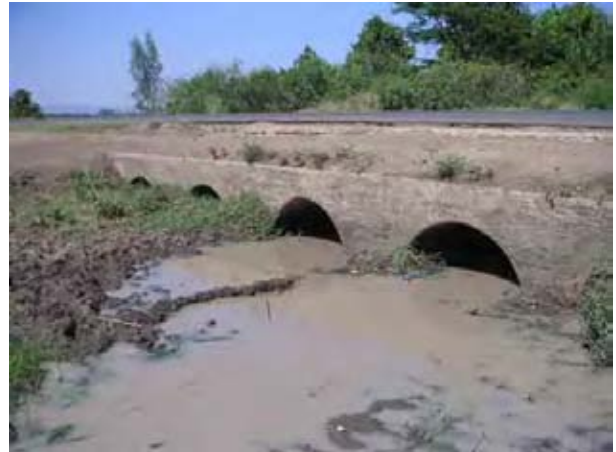
Plate 5 Culverts buried with sand.
