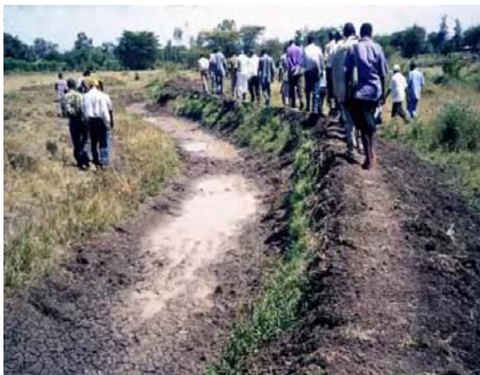
Plate 14: A cut-off drain to reduce flooding
