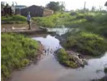
Clearing of blocked channels.
