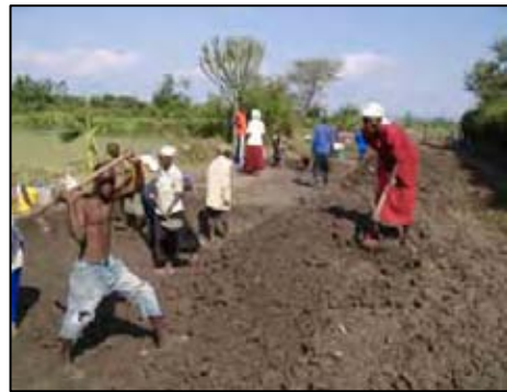
Rehabilitation of community road
