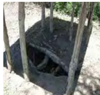
Sealing off all collapsed latrines.
