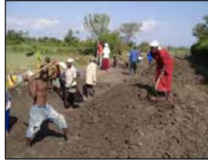
Rehabilitation of community road
