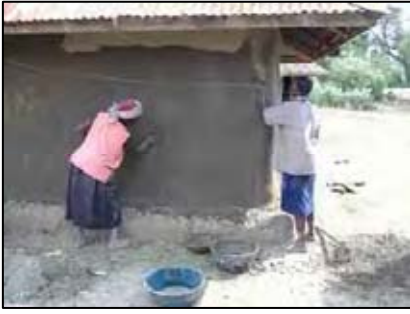
Rehabilitation of damaged house wall
