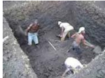
Digging of new latrines
