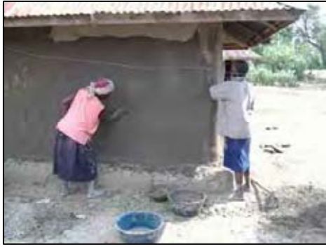
Rehabilitation of damaged house wall
