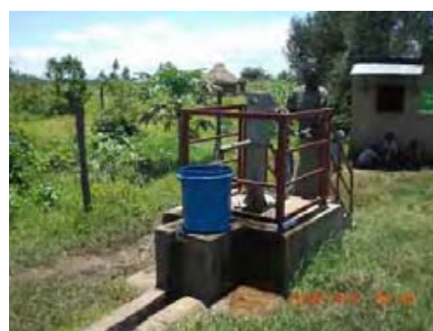
Completed Raised Well
