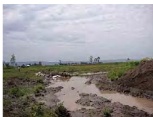
Damaged Dyke on Right Bank
