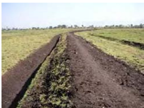
Sodding of Embanked Slope
