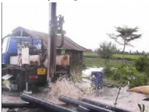
Drilling work in progress
