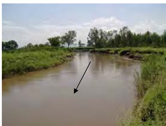
Lower Nyando near damaged dike
