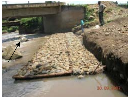
Completed Wooden and Gabion Mattress at Chil Chila Source: JICA Study Team
