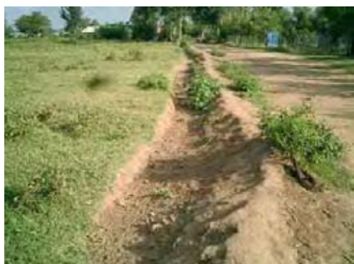
Draining Improvement in Odesso
