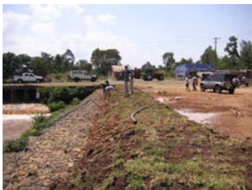
Sodding and Formation Works of the Dike at Odesso
