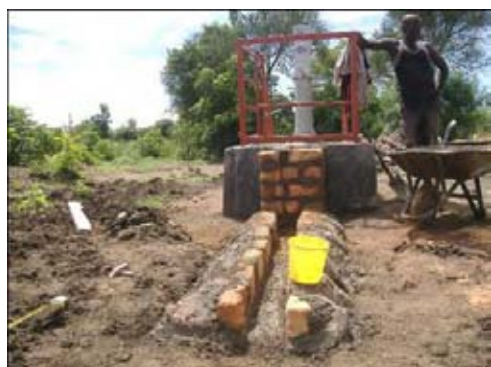
Construction of Additional Slab and Drainage
