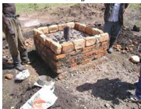
Construction of Slab
