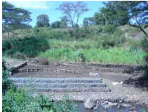
Bank Protection Works Constructed at Chil Chila
