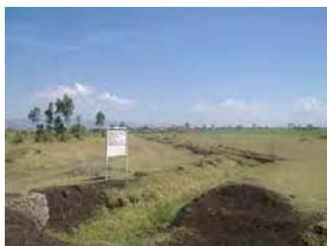
Extension of Raised Road by CBO in Kasiru
