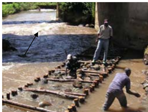
Wooden and Gabion Mattress in Progress at Chil Chila
