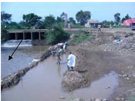
Coffering Works at Odesso
