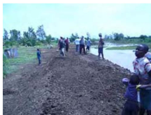
Embankment Works at Kochiewo
