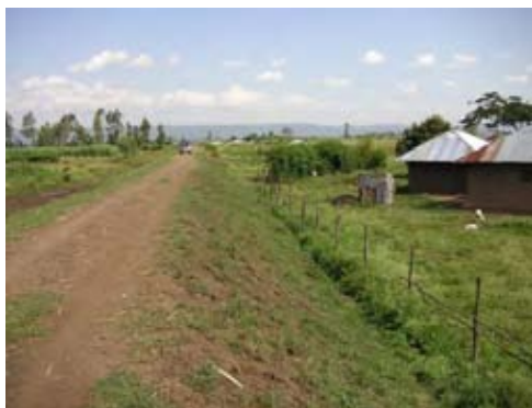
Rehabilitated Earth Dike (Landside) at Kochiewo
