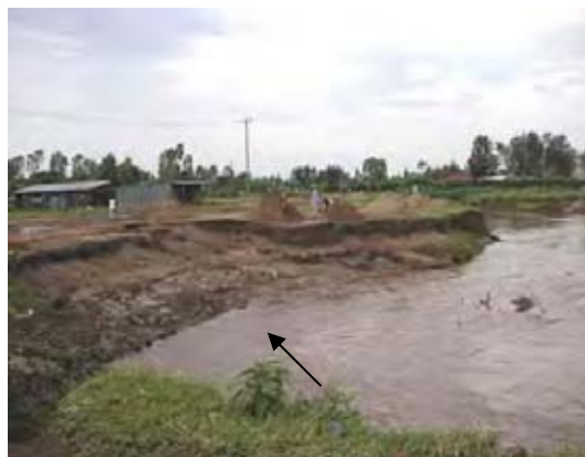
The riverbank greatly eroded by the flood
