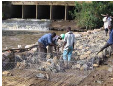
Fabricating Mattress for Gabion(1st layer) at Odesso
