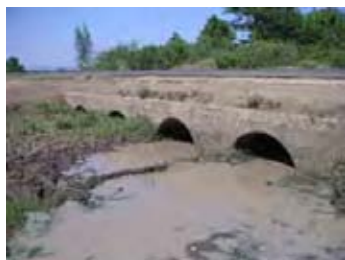
Bridge-7: Awach Kano Tributary
