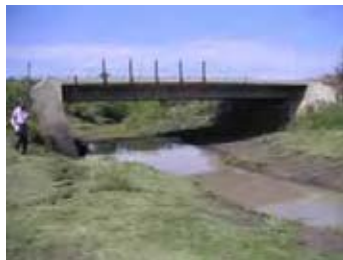
Bridge-2: Luando River
