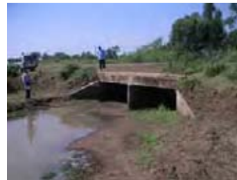
Bridge-3: Ombeyi River
