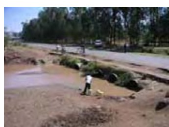
Bridge-8: Awach Kano River
