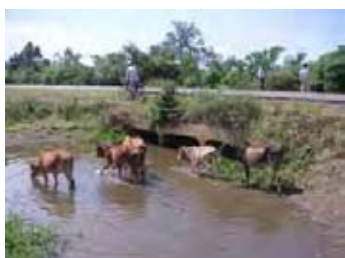
Bridge-4: Miriu River
