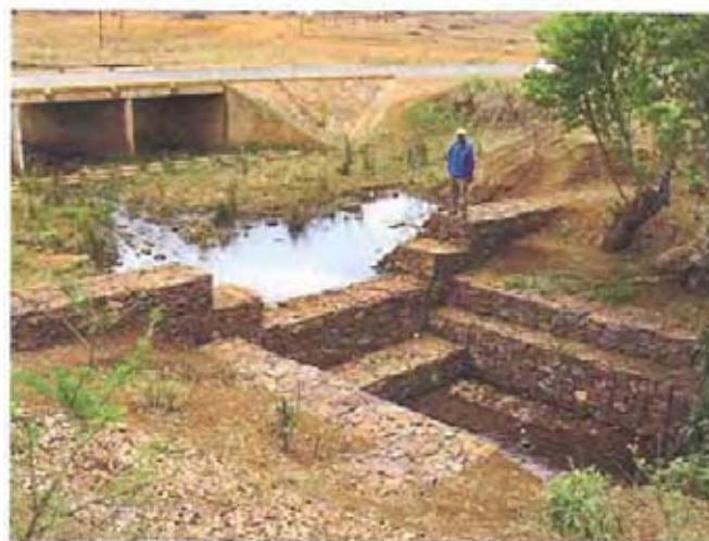
Figure 5.4.22 Example of Slit-type Weir
