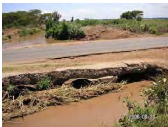
Culvert under A1 Trunk Road (Awach Kano R.)
