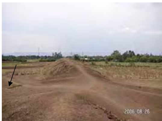
Dyke on Left Bank of Nyando
