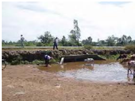
Culvert under A1 Trunk Road (Miriu R.)
