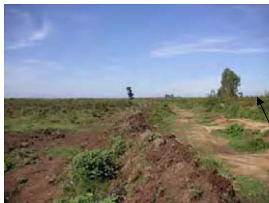
Dyke on Left Bank of Nyamasaria
