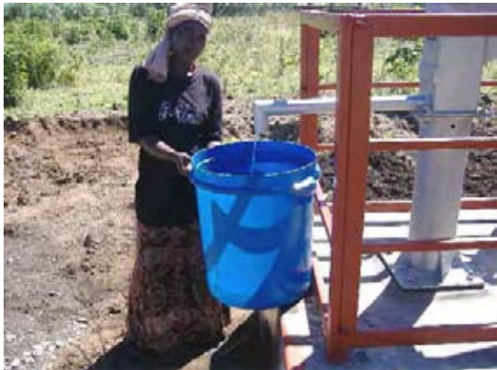
13. Completed handrail and hand pump
