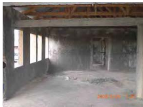
12. Construction of the inner wall
