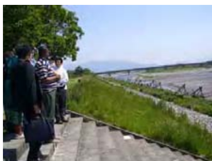
Inspection of Shingen Bank Facilities 1
