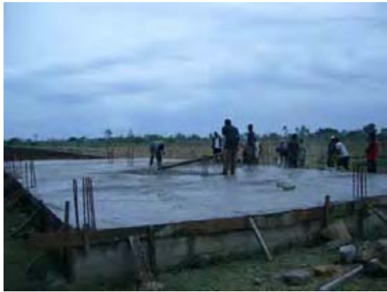
7. Concrete work at base part
