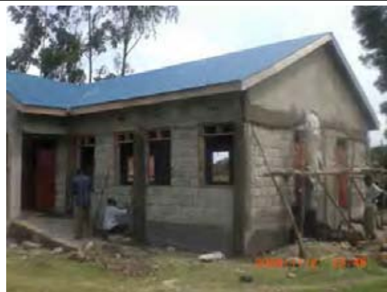
11. Construction of the outside wall
