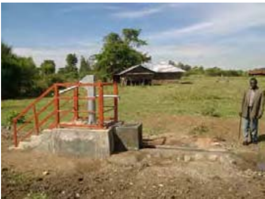
17. Completed raised well
