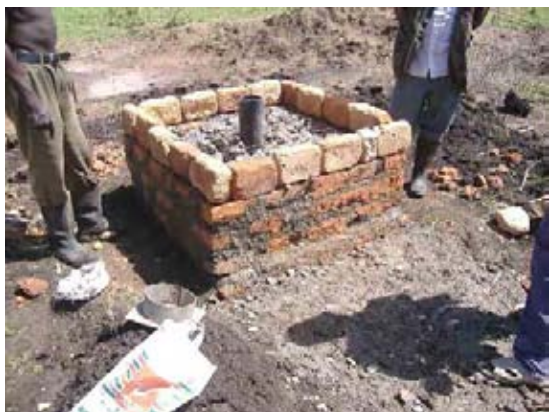
9. Construction of raised slab
