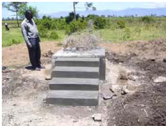
10. Completed raised slab
