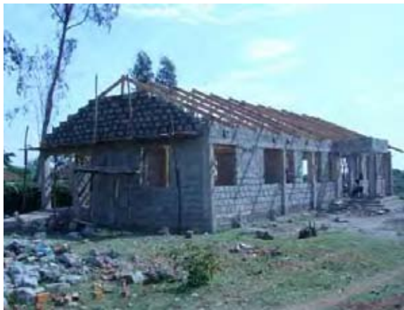
9. Construction of roof
