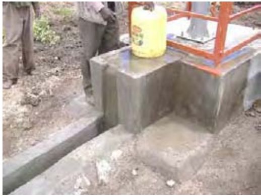
16. Completed raised well
