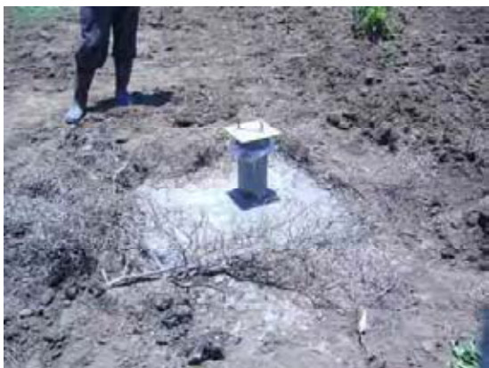
7. Completion of casing
