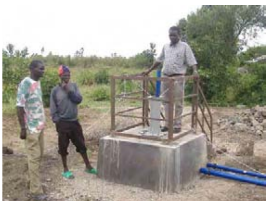
11. Installation of handrail
