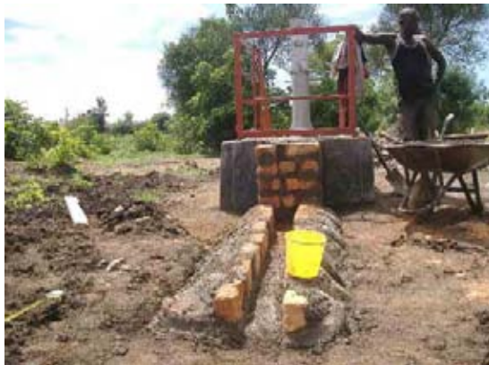
14. Construction of additional slab for bucket and drainage
