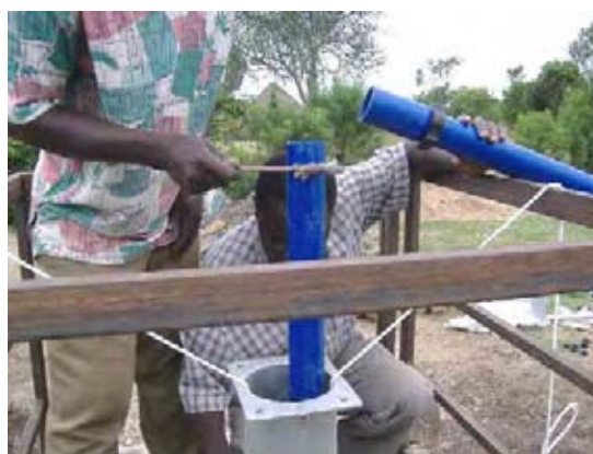
12. Installation of hand pump
