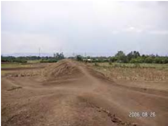
(a) Dike System along Nyando River
