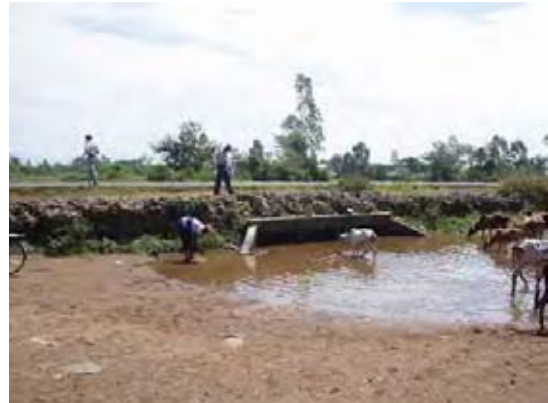
(b) Culvert at A1 National Road
