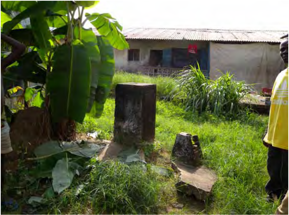
Existing Control Station RAMROD
