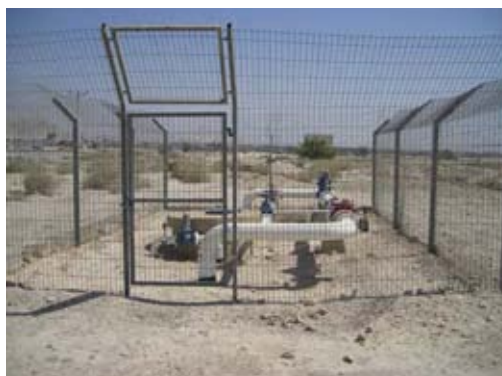
Connection Point of Mekorot Pipeline (as of July 2008)
