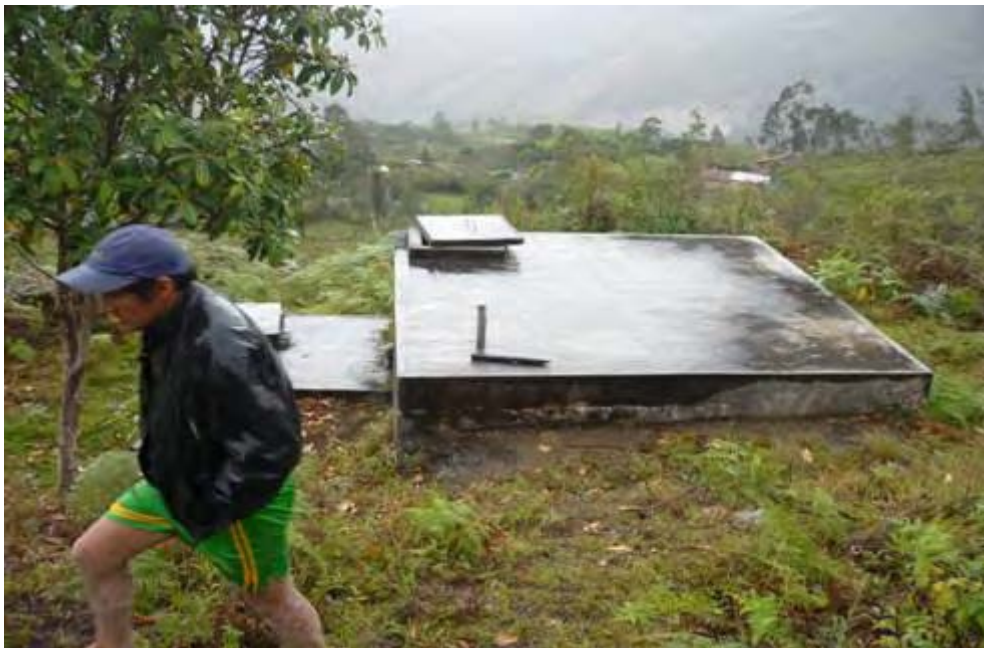
Rectangular Reservoir of 20 m 3 - Cocachimba
