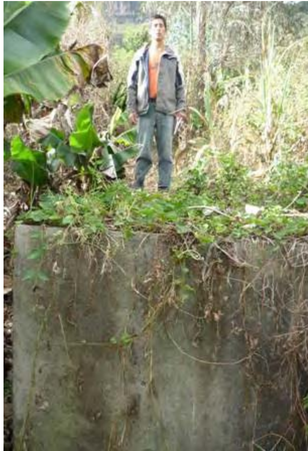
Septic Tank - San Pablo
