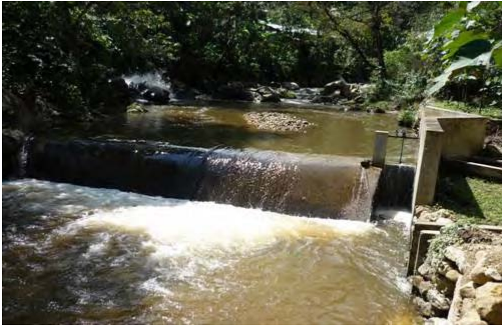
Catchment on the Ingenio River – Second Sistema
