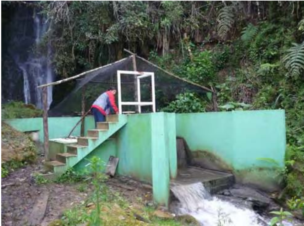
Catchment at the Ollapata Gully – San Carlos
