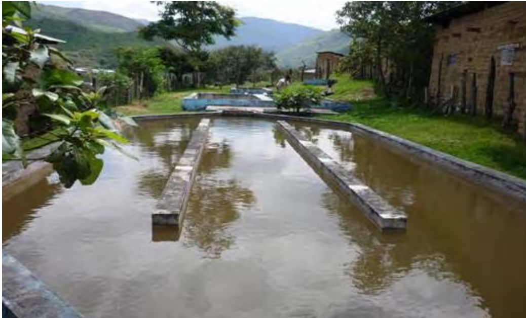
Treatment Plant – First System – Main view of the Storage Unit
