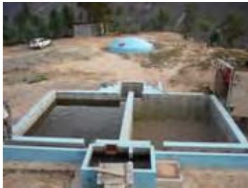
Slow Filter for water treatment in Magdalena
