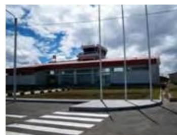
New terminal entrance
