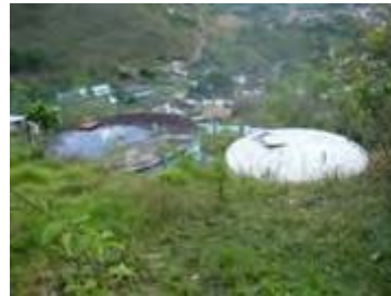
Reservoir tank in Leymebamba
