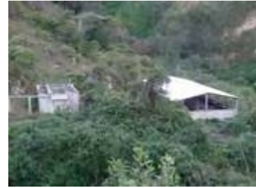
Imhoff type Tank for sewerage treatment in Leymebamba
