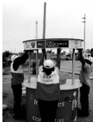
Photo: Kiosk installation, Independencia. October 2008.
