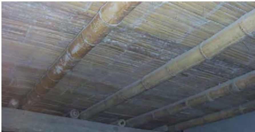
This roof shows the Guayaquil canes and over it the crushed cane
