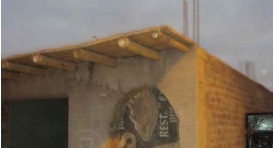
The roof of this house shows the Guayaquil cane, the crushed cane and the mud cake
