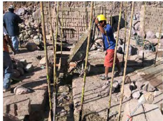
Casting of concrete for foundation
