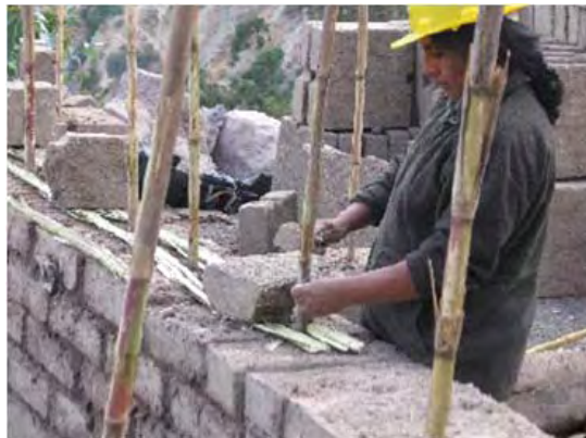
Vertical canes for reinforcement
