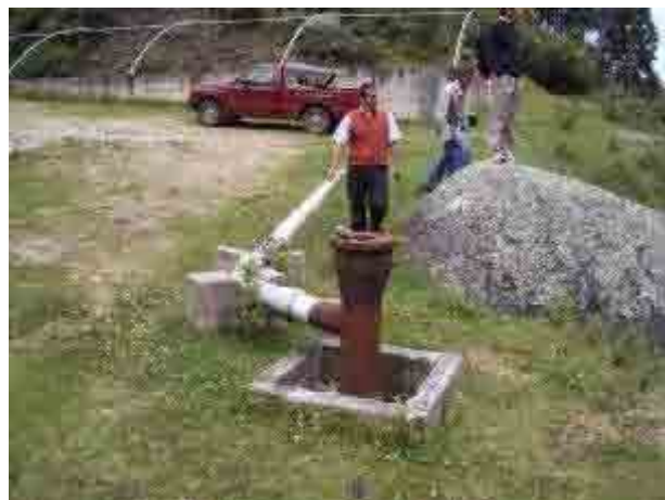
Photo-2 Pilot Project site (Acueducto well)
