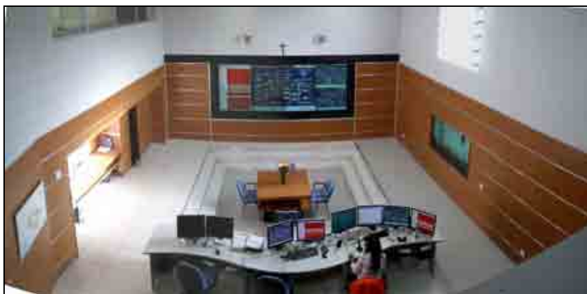
Figure-2.1- 36 Picture of Central Control Room at Central Control Center
