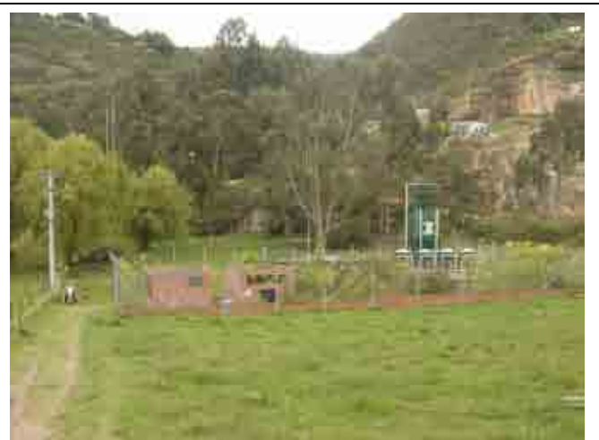
Water treatment facility for groundwater in Tocancipa. Proposed facilities for water treatment in this JICA Study is more compact than this.
