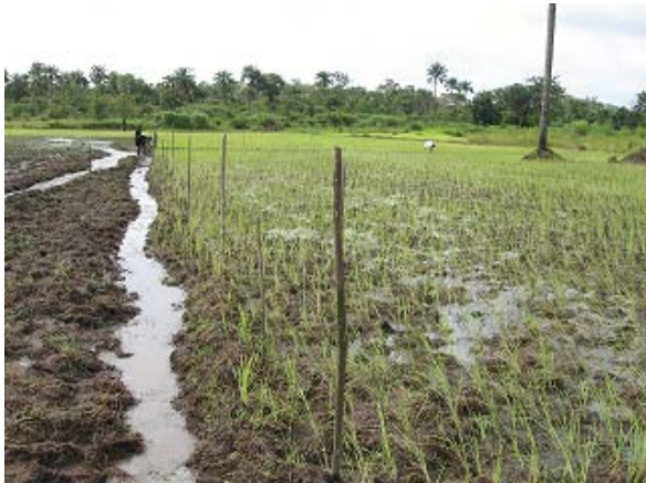
Photo 2.5-6 Bund Constructed along Drainage Channel
