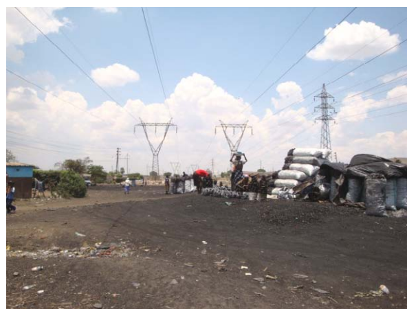
Illegal Charcoal Market in Misisi Compound under Transmission Lines Photograph: JICA Study Team
