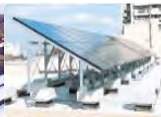
Small Scale Solar Panel Use
