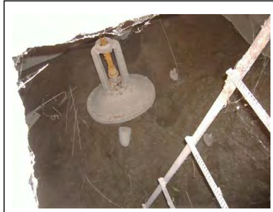
Inside of Dzhilikul - Grauti Junction Valve Box
