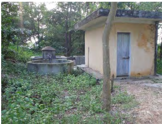
Leachate treatment facility
