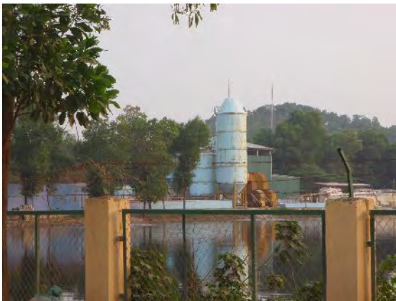
Leachate treatment facility
