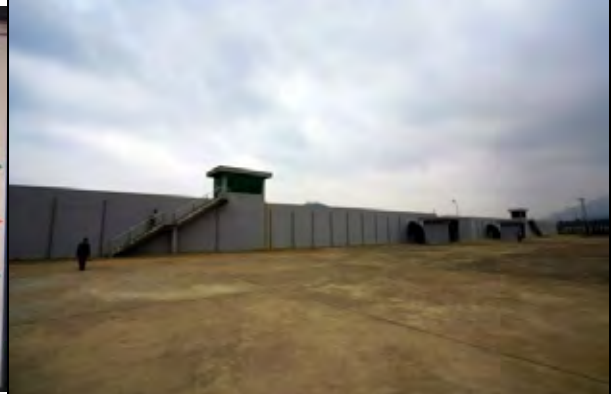
Photo 10: Da River Water Supply Project Hoa Binh Treated Water Reservoir with capacity of 60,000m 3
