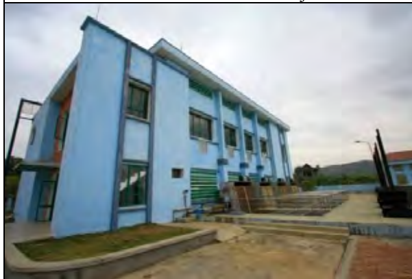
Photo 3: Da River Water Supply Project Intake Pumping Station
