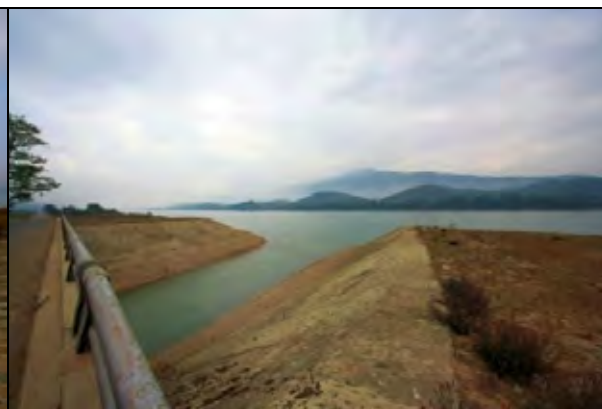
Photo 2: Da River Water Supply Project Intake Structure
