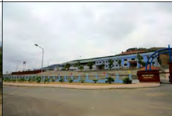
Photo 6: Da River Water Supply Project Water Treatment Plant with capacity of 300,000m 3 /d
