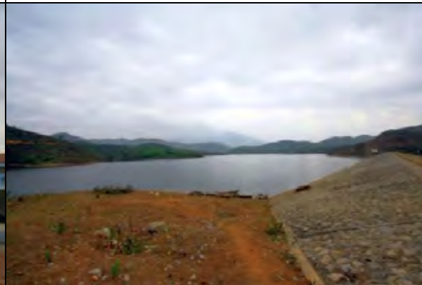
Photo 4: Da River Water Supply Project Lake as a raw water reservoir
