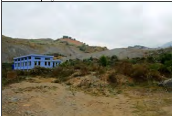
Photo 5: Da River Water Supply Project Lift-Up Pumping Station from reservoir to plant
