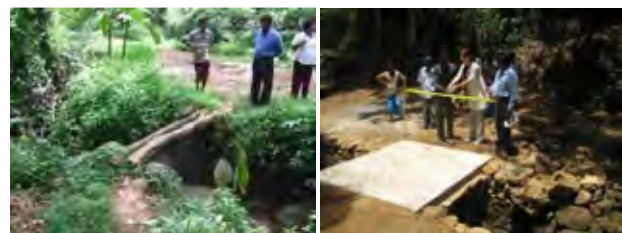
Kiribathgala project site: Crossing- before (left) and after (right)
