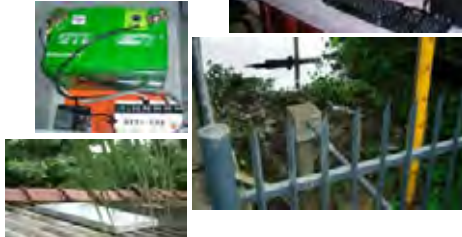
Water level gauge at Nagalagam St., Battery and Data Logger, Solar Panel (Left October, 2007)
