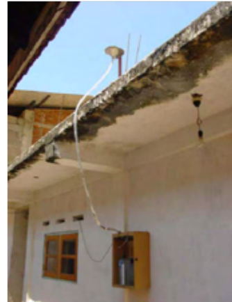
Installed rain gauge
