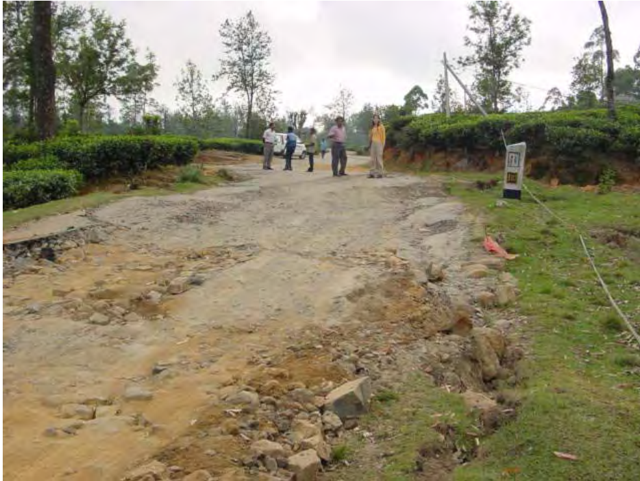
Figure N.2.11 Landslide at the Estate in Diyan Hawatta
