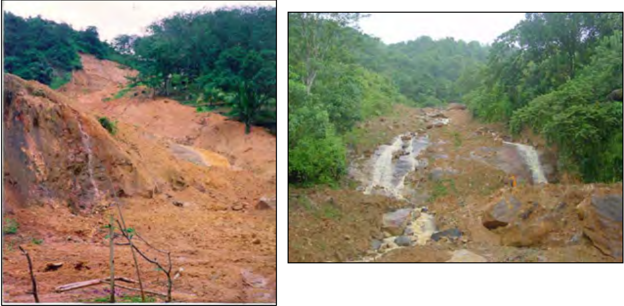
Figure N.2.5 Earthflow at Helauda (left: photos by NBRO in 1994, right: in 2006)
