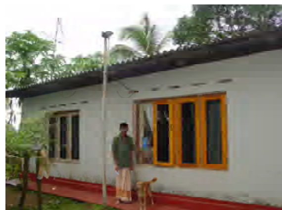
Installed rain gauge
