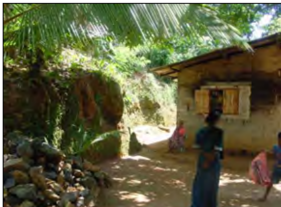
cutting slope behind the house
