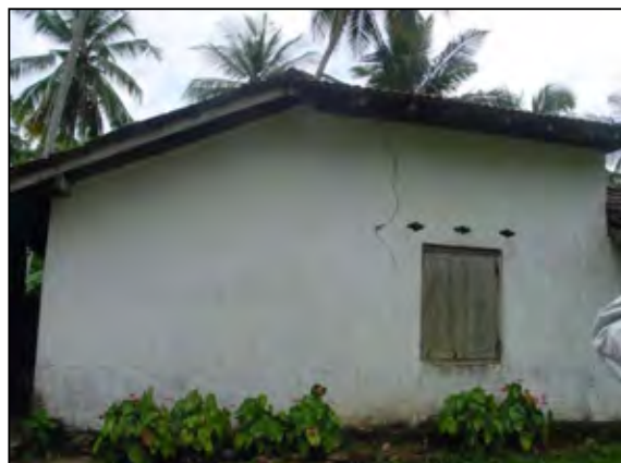
crack on the wall
