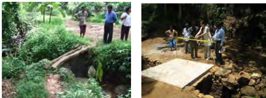
Figure M.4.16 The crossing before improvement (left)/ the constructed crossing (right)
