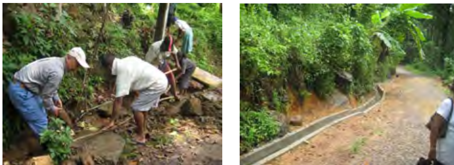
Figure M.4.14 Cleaning of the Drainage Canal (left) / The Improved Drainage Canal
