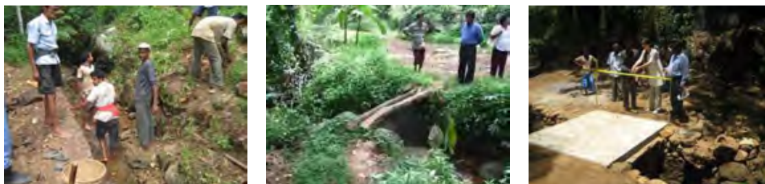
Figure IV-20 Construction Work/ Crossing before improvement (center)/ after improvement (right)
