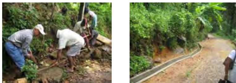
Figure IV-19 Cleaning of the Drainage Canal (left) / The Improved Drainage Canal
