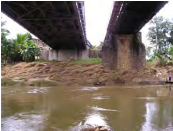
Steel Truss Bridge in Ratnapura (WL G/S is operated)
