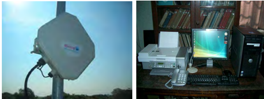
Figure III-12 Installed Equipment (Antenna for Wimax (Left), Provided Equipment for each organization (Right))
