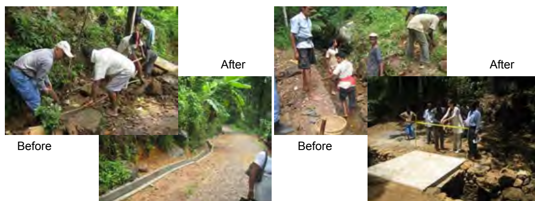
Figure 30 Drainage Canal Rehabilitation (left)/ Construction of Evacuation Crossing (right)
