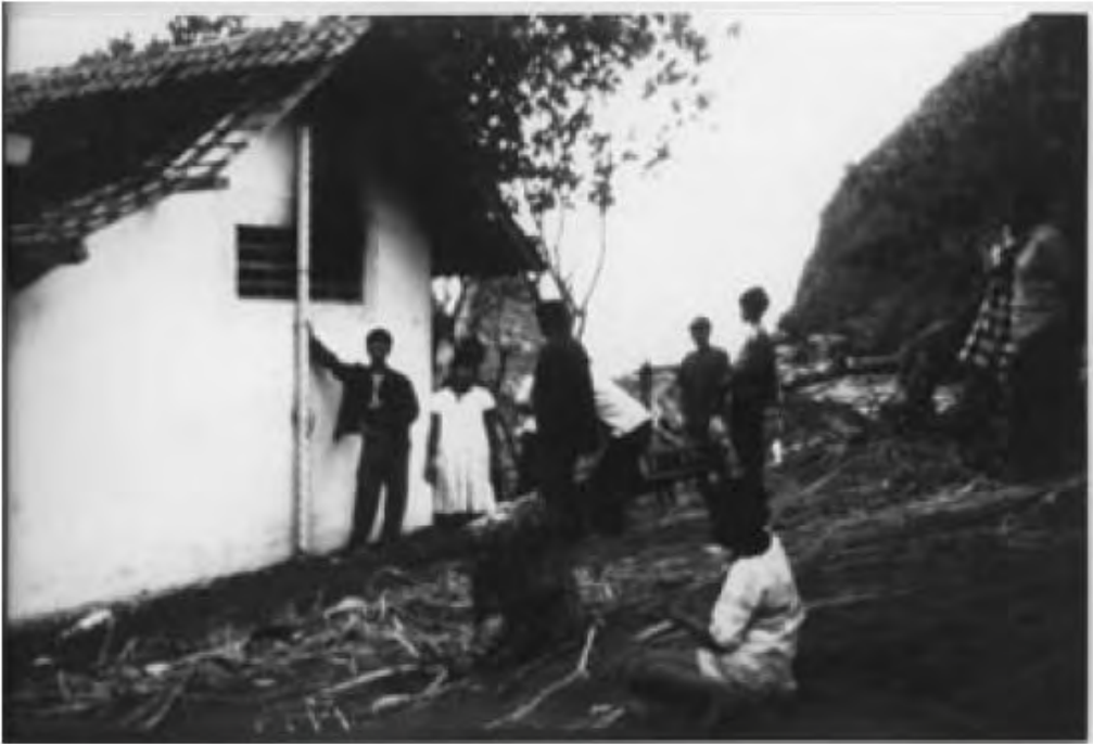
Figure 7. Watuulo: damaged house where marks of three different waves were observed. The third wave caused the roof collapse.
