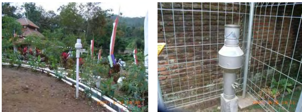
Figure 5.2.2 Rain Station in Plantation Area (left); Irrigation Department Rain Station (right)
