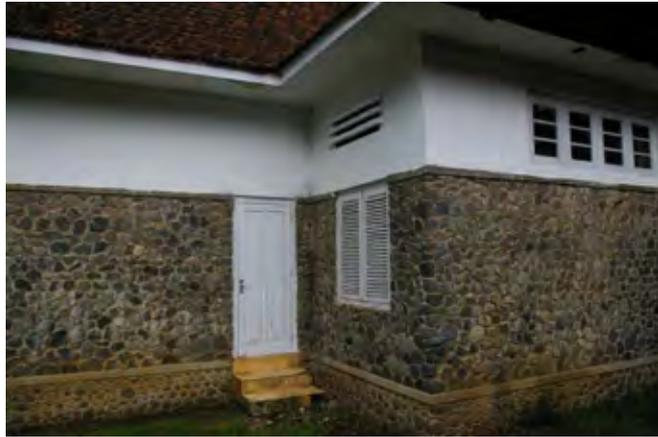
**Figure 3.1.18 Cobble Masonry**
