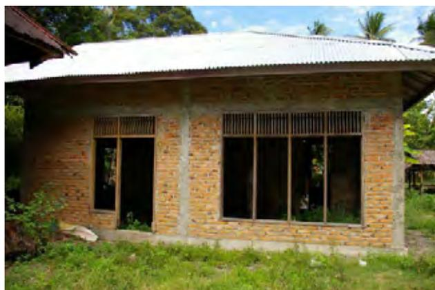
**Figure 3.3.23 Confined Masonry**
