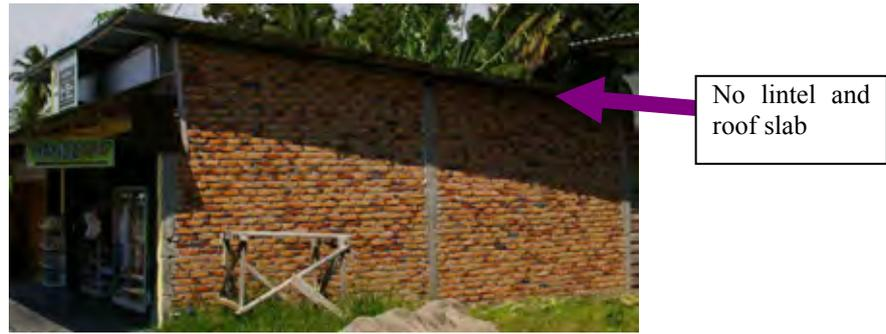
**Figure 3.2.27 Building with no Lintel and Roof Slab**
