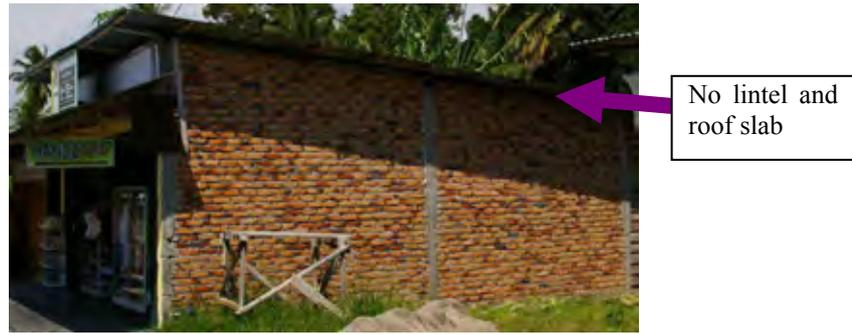
**Figure 3.1.22 Building with no Lintel and Roof Slab**
