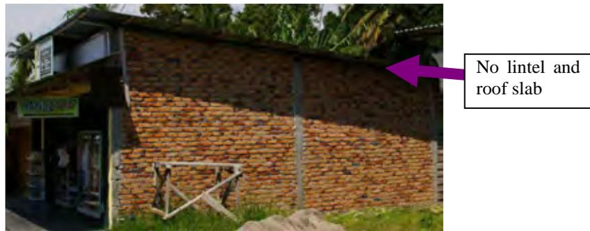
**Figure 3.3.26 Building with no Lintel and Roof Slab**
