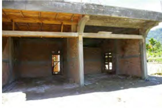
**Figure 3.3.24 Reinforced Concrete Moment Resisting Frame**
