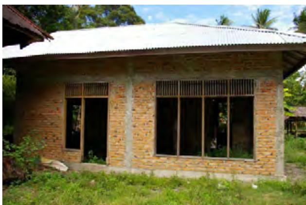
**Figure 3.2.24 Confined Masonry**
