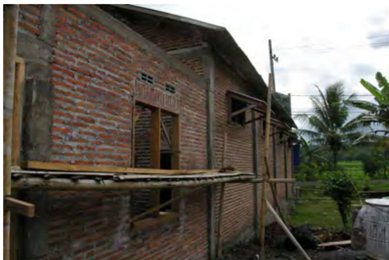
**Figure 3.1.19 Confined Masonry**
