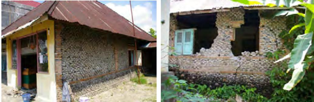
**Figure 3.3.22 Cobble Masonry**
