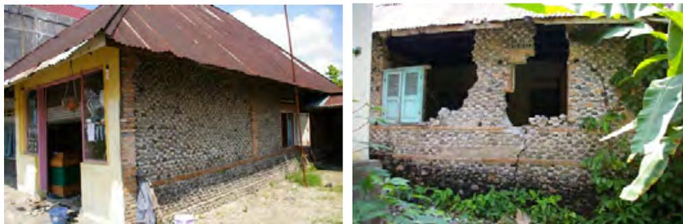
**Figure 3.2.23 Cobble Masonry**
