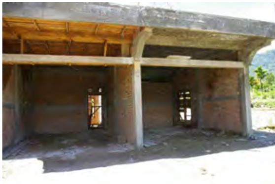
**Figure 3.2.25 Reinforced Concrete Moment Resisting Frame**
