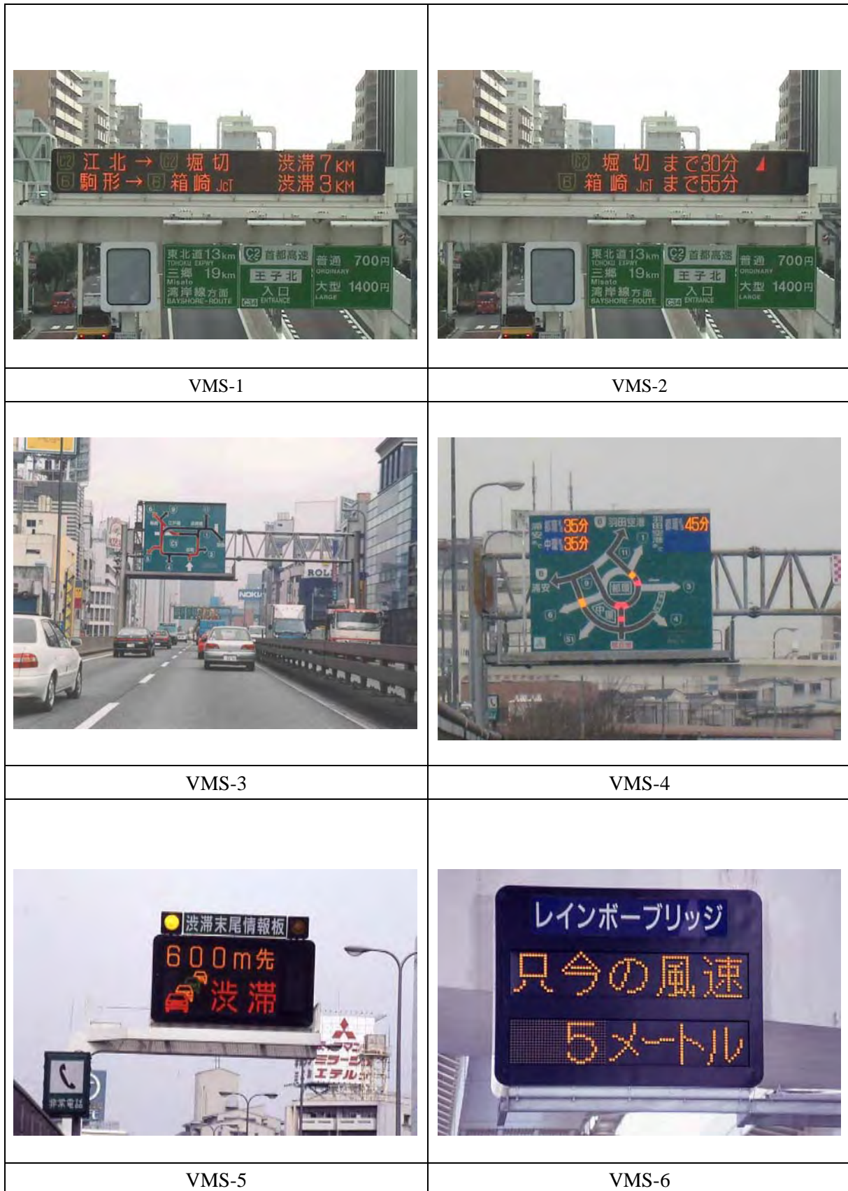
Figure 9.4-12 Example of Variable Message Signs in Tokyo Expressway
