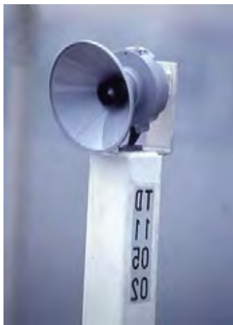
Figure 9.2-8 Ultra Sonic Vehicle Detector Head
