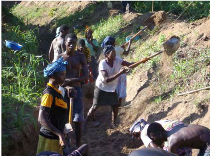
Pilot project: Participation of beneficiaries in irrigation canal rehabilitation (Canjala Comuna )
