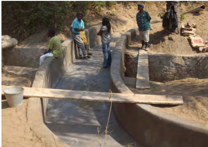
Pilot project: Rehabilitated portion of canal (Canjala Comuna )
