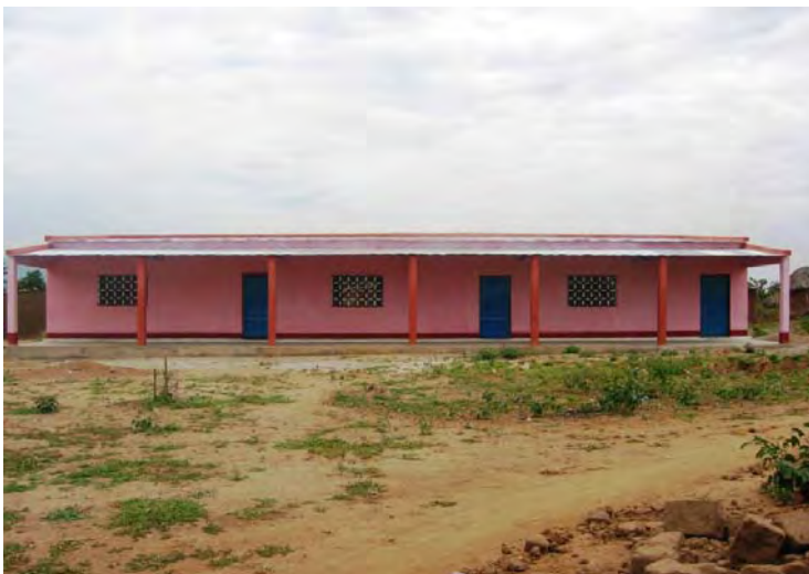
Pilot project: Constructed school building (Canjala Comuna , Kateque village)
