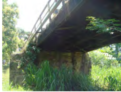
Bridge No. 1 (240/4 橋) の桁下
