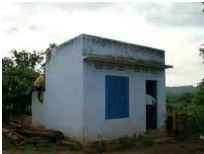
<P-6 Ea Cha Rang> Deep well and Pump house
