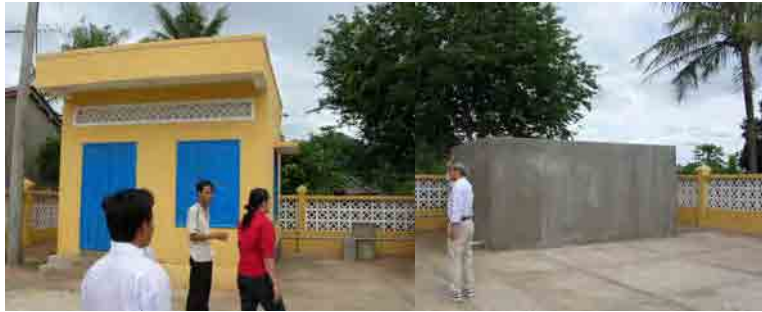
<P-5 Son Phuoc> Water treatment plant
