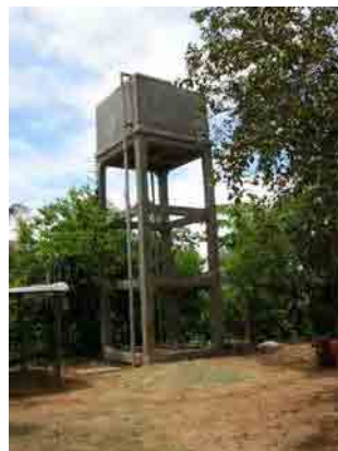
<K-1 Cam An Bac> Elevated tank
