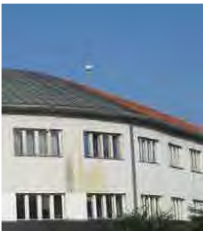
Photo 14 : GPS-based reference station on the roof of Pljevlja city office
