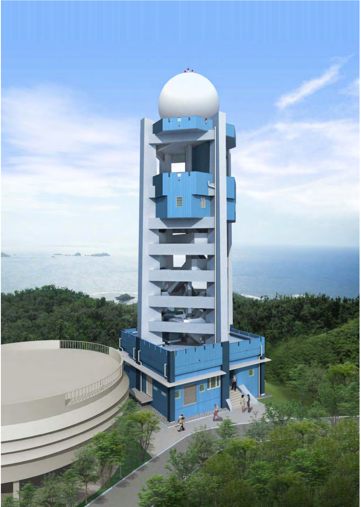
Virac Meteorological Radar Tower Building
