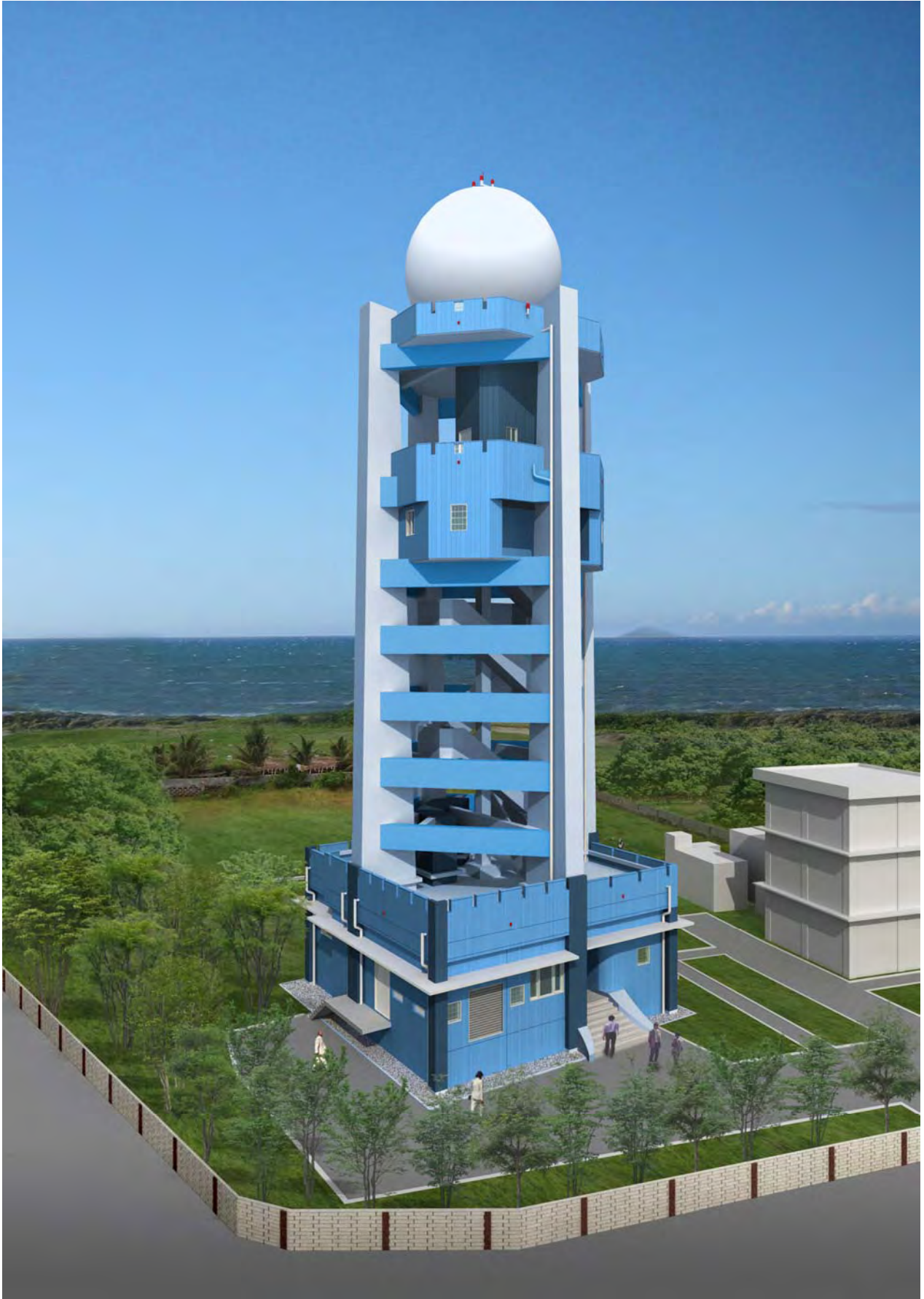
Aparri Meteorological Radar Tower Building
