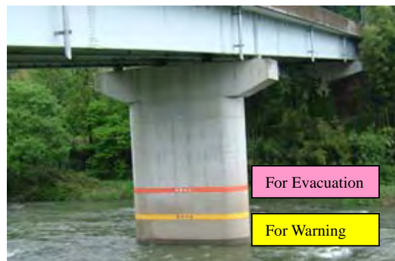
Photo-8 Example of River Water Level Indicator for Flood Warning and Evacuation
