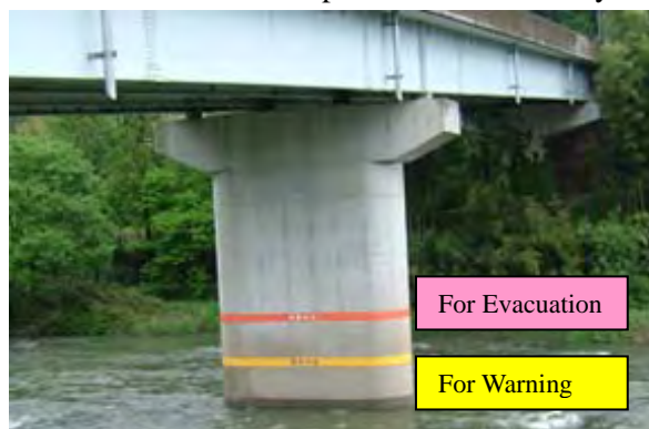
Photo-1 Example of River Water Level Indicator for Flood Warning and Evacuation
