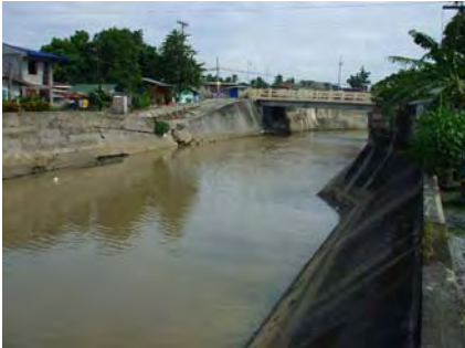
Fig. R 2.7 Dike Failure of San Juan River
