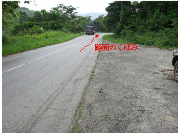
写真-3：路面のくぼみ
