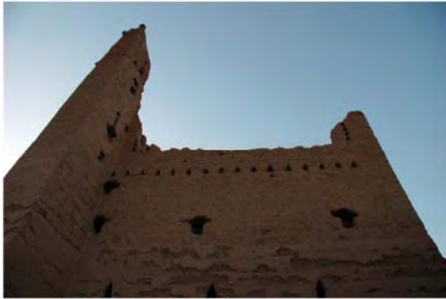
Figure AP4-1.54 Adobe Structure near Riyadh
