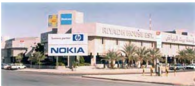
Figure AP1-51 Al-Jeraisy Group Office Building
