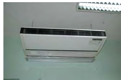
Figure 7- 50 Ceiling Fan of Air Conditioner
