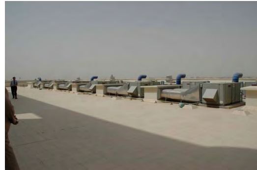
Figure 7-61 Roof of MOWE Building
