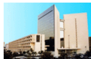
Figure 7-46 King Faisal Foundation (KFF)
