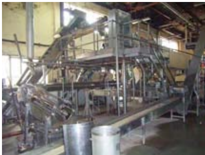
Sanitary processing line in Parwanoo plant.
